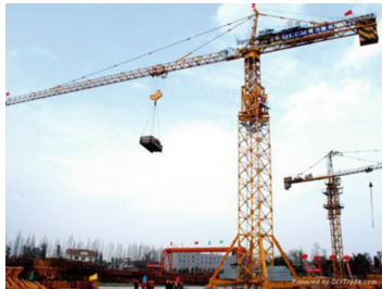
FIGURE 1 – Tower Crane in Construction Site [1]
